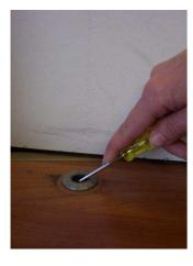
The Floor Sockets fitted are an important part to the locking of your store. Should they become damaged or blocked with debris, the locking mechanisms may fail to engage preventing you from securing the store after closing.
